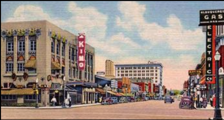
Looking East from Fifth Street & Central Avenue
